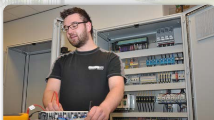
Control panel building
